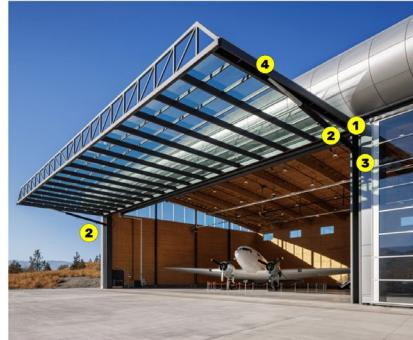
High quality single-panel hydraulic doors, like PowerLift offers, consist of a structural stationary frame and a one-piece door leaf that is hinged at the top of the frame. The PowerLift door system arrives fully assembled in one piece and is attached to the building opening. The door system opens using two hydraulic cylinders powered by an electro-hydraulic power unit.
